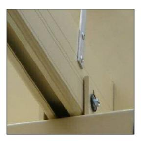
2. Site the adjuster mechanism in a position which allows you easy access and ensure that the opening and closing handle will be in a convenient position for you.
