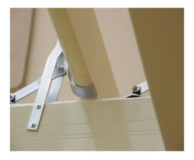
8. Use a normal pair of pliers or footprints to crimp the louvre clip to the louvre as shown.
