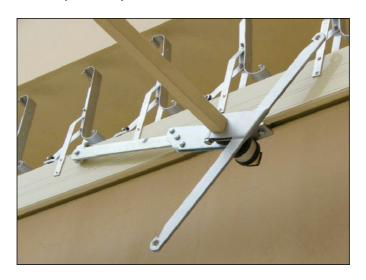
7. Slot the louvres into the louvre clips and clip home as shown in the video.
