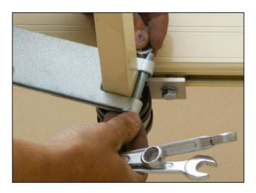
6. Fit the opening and closing handle to the opening and closing bar with the bolt provided. Once fitted fully open the louvre clips so they at 90° to the louvre beams.
